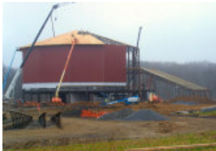
Closeup of the construction (Photo: Gettysburg Foundation)
