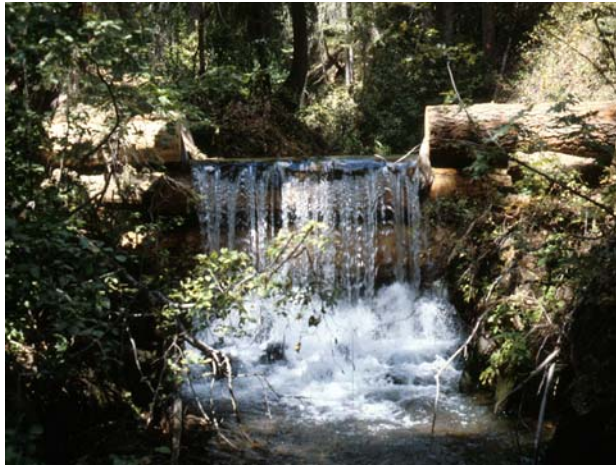
Figure 11. Fish barrier constructed primarily of natural materials. (Photo courtesy of Mark Buktenica, Crater Lake National Park.)
