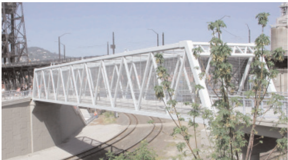
Bridge over Union Pacific tracks. Portland, OR
