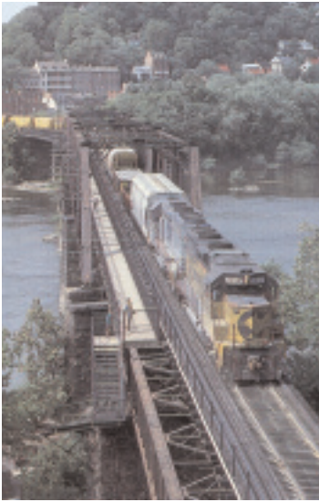
Harpers Ferry Bridge. Harpers Ferry, VA
