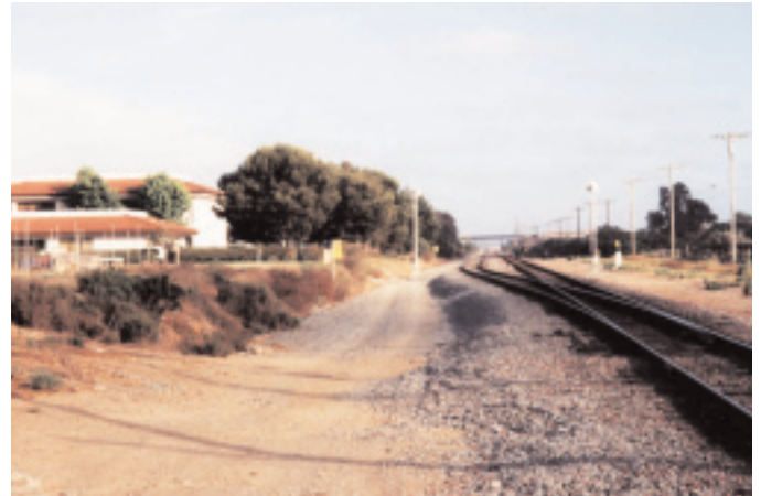
Future trail alignment of the Coastal Rail Trail extension adjacent to the Coastline tracks. Carlsbad, CA
