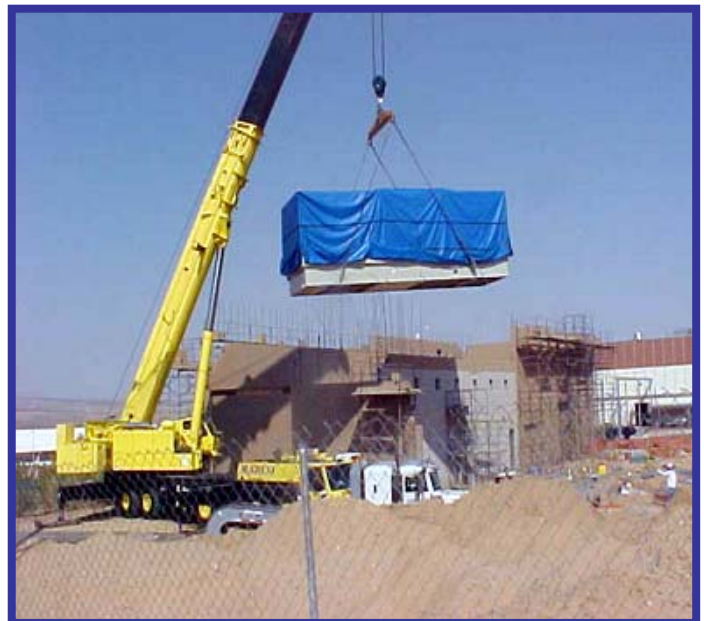
CHP plant under construction; lowering the turbine into the turbine hall.
