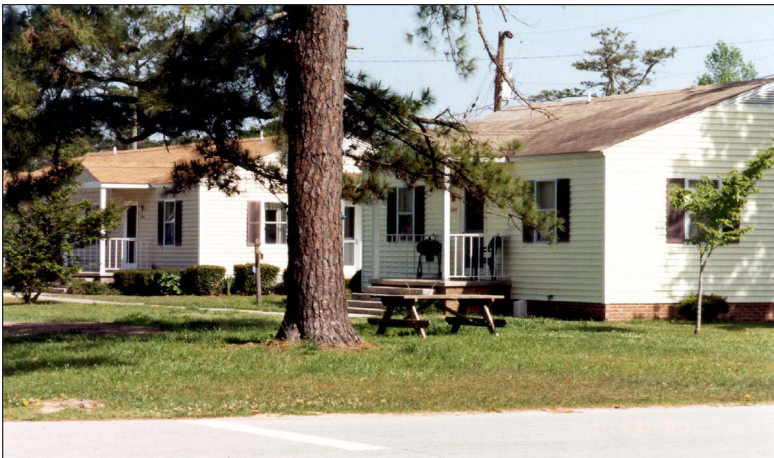
Almost half of Camp Lejeune's 4477 family housing units were retrofitted with GHPs.
