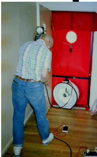
Comprehensive weatherization utilizes blower doors and other advanced diagnostic and implementation techniques.
