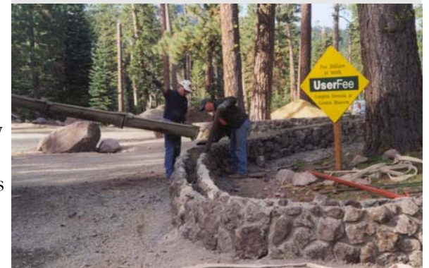
Loomis Museum Plaza Renovation
