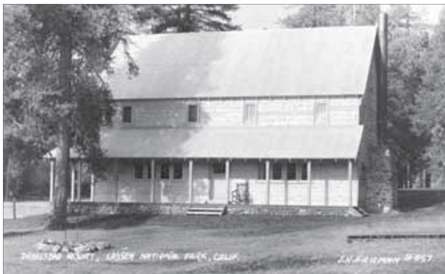
Photograph showing the porch along the east façade of the new lodge building, rebuilt by the Sifford's in 1938 after a winter snow storm that demolished the original lodge. Photo, 1938. (LAVO Collection, DB26)
