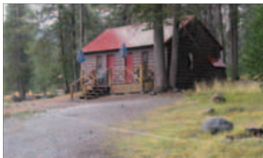
Contemporary view looking southwest toward the Duplex Cottage. Photo, 2003. (National Park Service)
