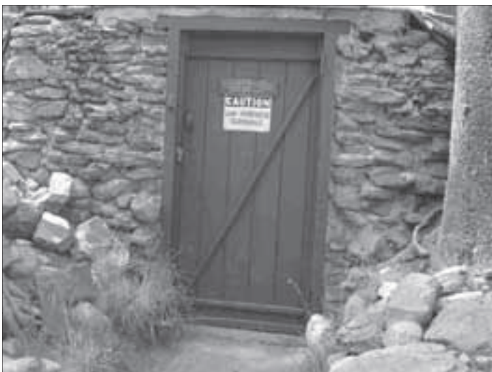
Contemporary view of the food locker (HS-3). Built into the slope, this structure is believed to have been constructed in 1900 as a cold food storage facility. View looking southwest. Photo, 2003. (National Park Service)
