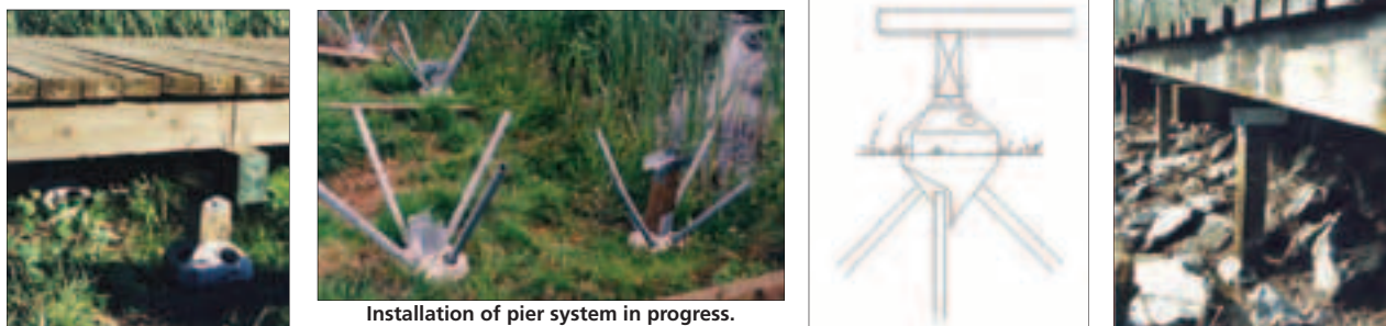
Photographs of the Pin Foundation Diamond Pier and boardwalk from the Nisqually National Wildlife Refuge.
