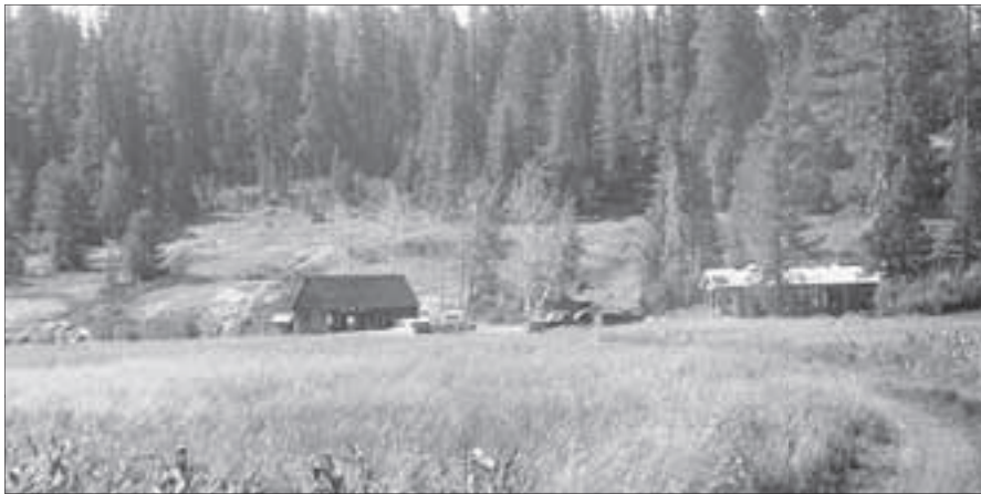
For a short time the swimming pool was flanked by two bath houses, east and west of the pool. This photograph shows the new bath house (on the right) under construction. Photo, 1962. (LAVO Collection, newbath)
