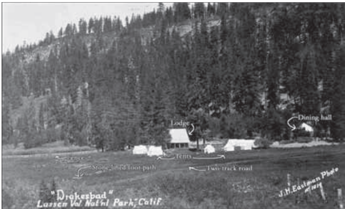
Early core development, including the lodge and the dining hall, was located north of the meadow. A fence system, stone lined foot-path, and two-track road are visible within the meadow. Photo, circa 1926. (LAVO Collection, Eastman photo #1014.)
