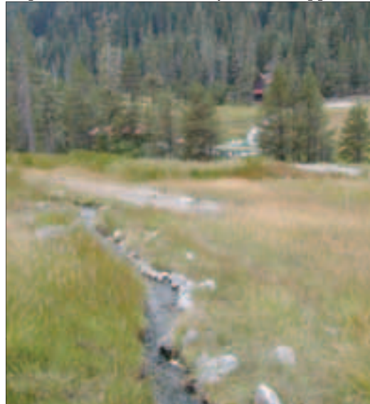
A rock lined earthen ditch, up slope and south of the pool, transports the naturally heated water to a conveyor box. Photo, 2003. (National Park Service)
