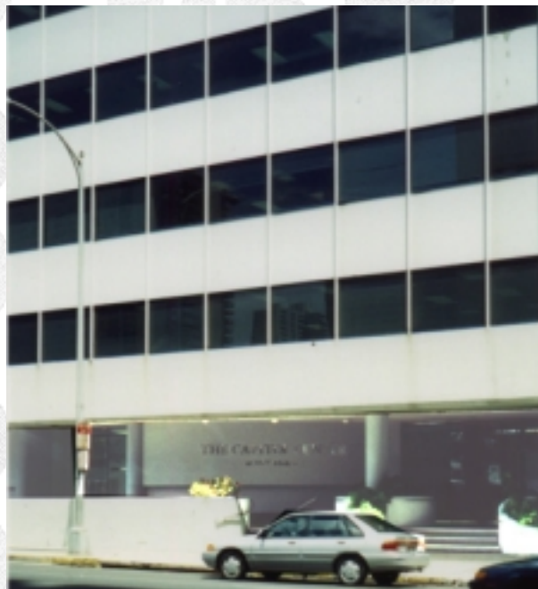
Capitol Center on Alakea Street: the Bureau's home during the Capitol
