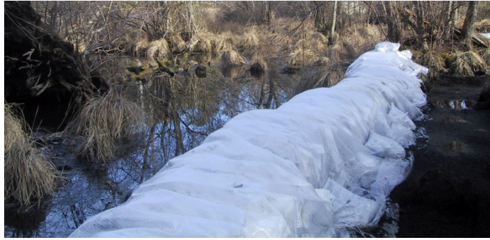
Area A: Sandbags cross the river at the site of the upcoming pilot study that will evaluate the vacuum guzzler technology. The sandbags help dry up the portion of the river slated for the vacuum guzzler study.
