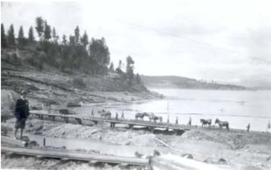
Construction work on Jackson Lake dam, Upper Snake River basin (Oct. 1914)
