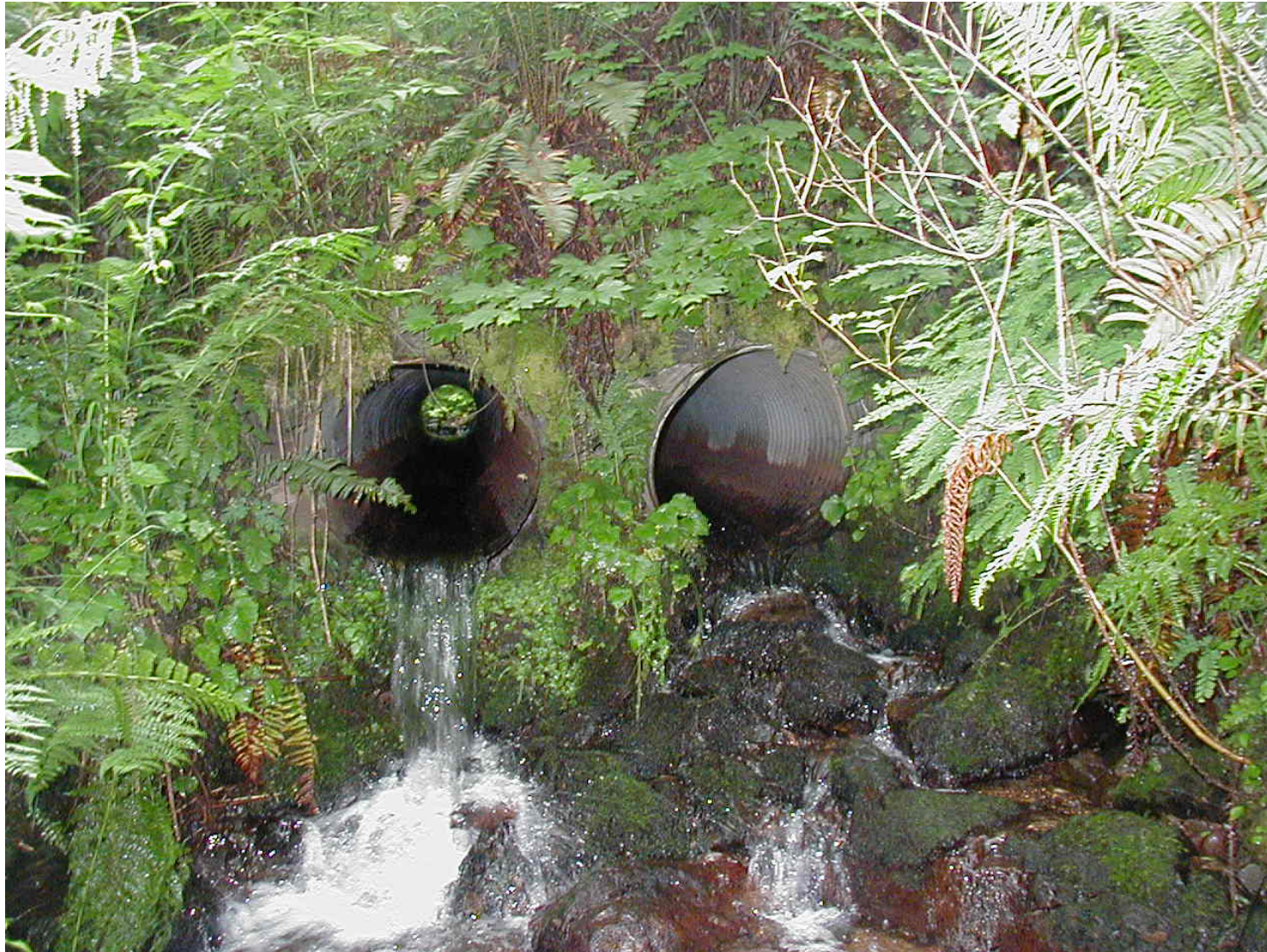
Figure 2. Outlet of double barrel culvert at milepost 21.1.
