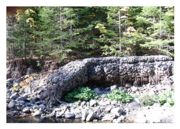
Figure 6. Failing gabions at Cabin 20.
