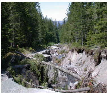
Photo: Flood Damage - Forest Road 81 near Kalama Horse Camp
