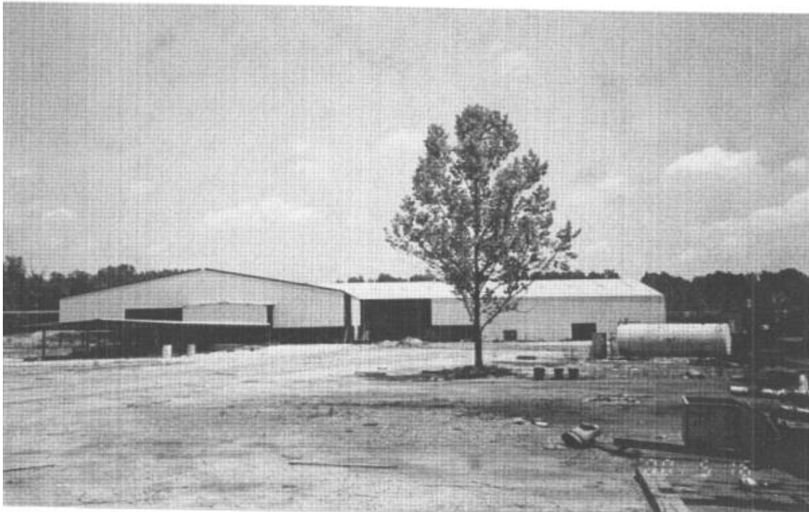
Exterior of Sawmill
