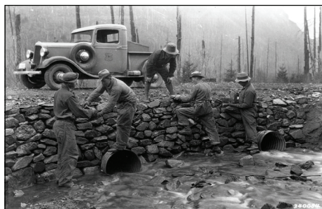
CCC crew on the Cispus Road.
