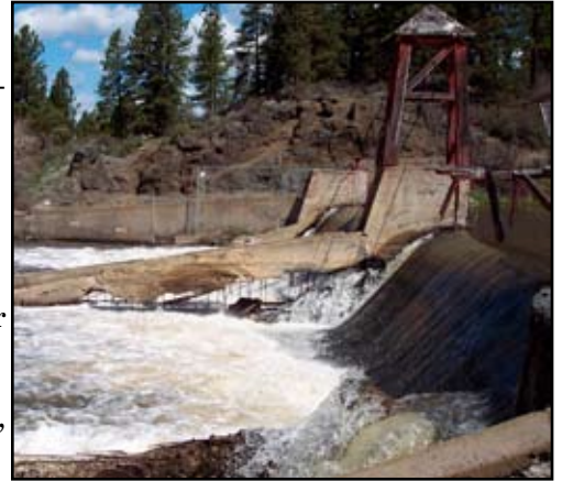
Built in 1914, Chiloquin Dam helped farmers in the Upper Klamath Basin irrigate their fields. Now irrigators will get water deliveries through a new pumping system. (USFWS photo)
