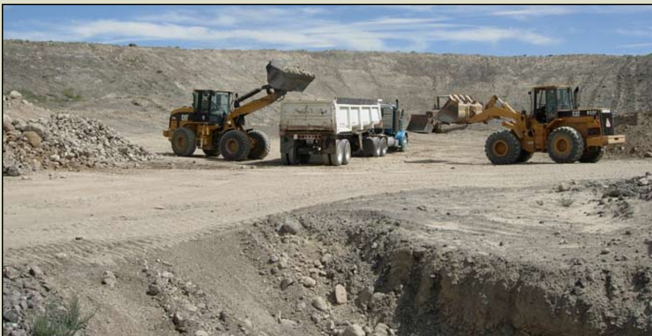
Working together to repair the breach. (Janet Schmidt/USFWS)
