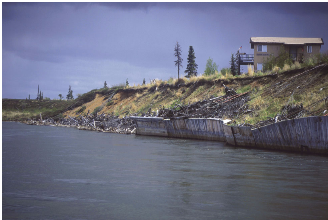
Figure 28. Trees and a revetment as erosion control, Alagnak River river kilometer 38. Photograph by author, June 7, 2001.
