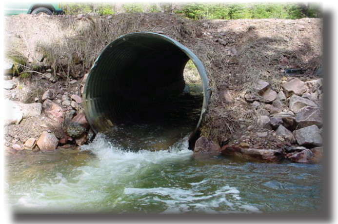
Lolo National Forest culvert - before replacement
