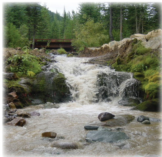
Rich Creek culvert after replacement. Kootenai National Forest
