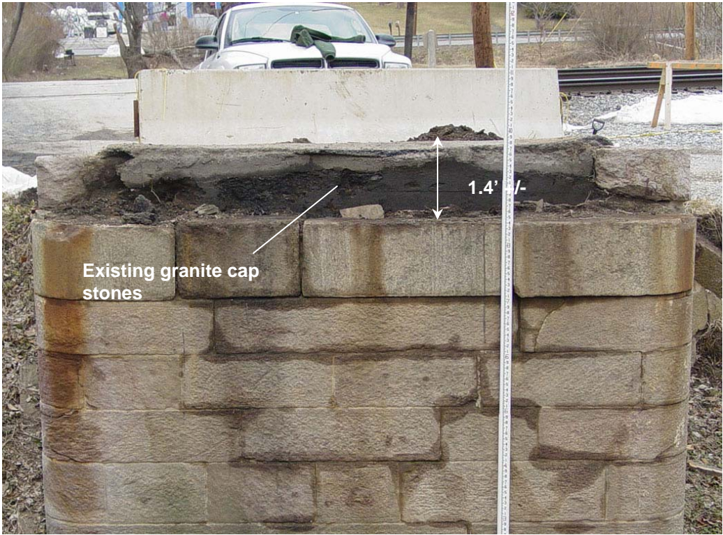
North abutment with steel super structure and bridge decking removed.
