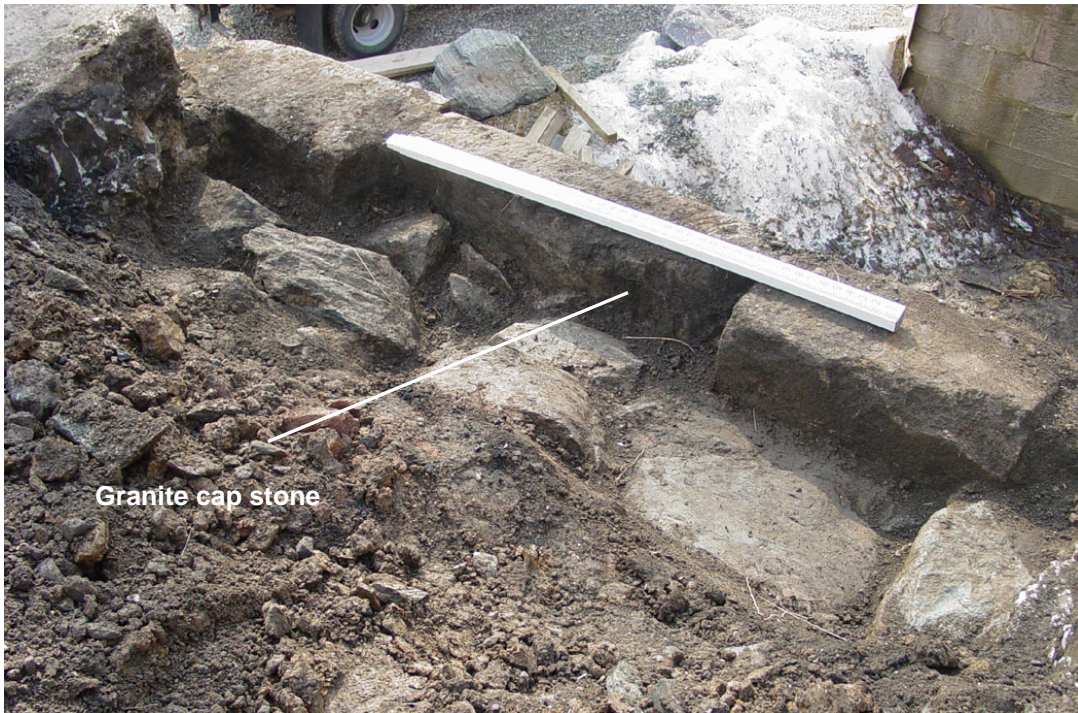
Excavation behind granite cap stones - North Abutment
