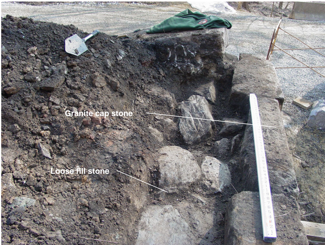
Excavation behind granite cap stones - North Abutment
