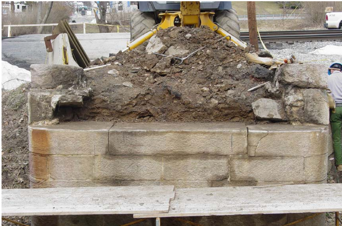
North abutment with granite cap stones removed.
