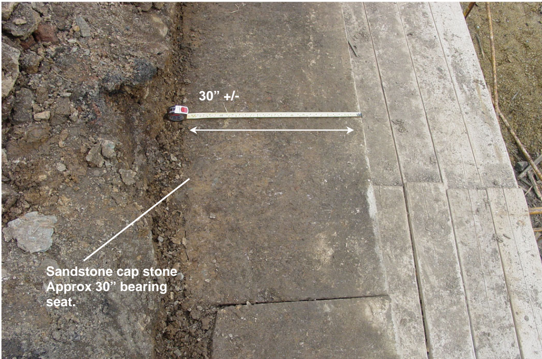
North abutment with granite cap stones removed.
