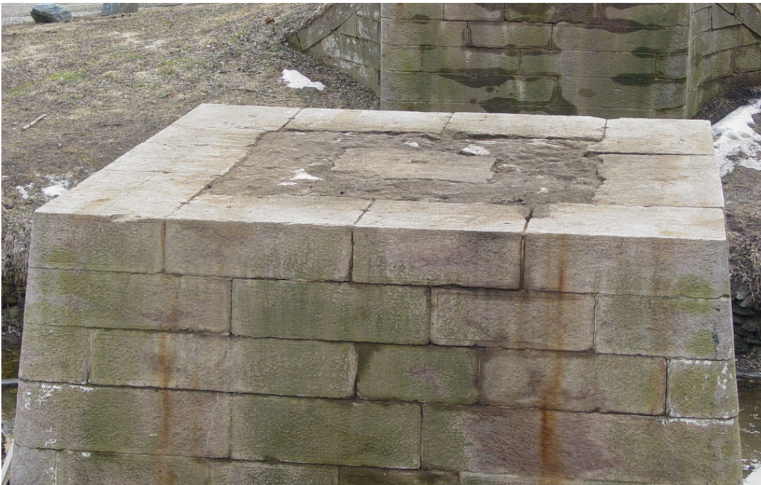
Center pier with steel super structure and bridge deck removed.
