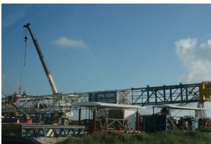
Kindie Oil & Gas setting up rig
