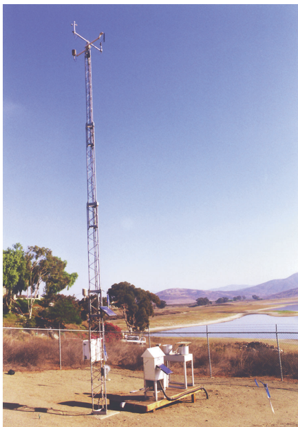
Figure 7. Air monitoring station at Sweetwater Reservoir.
