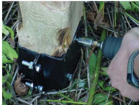
Above: Installing the Groundmaster Post System.
