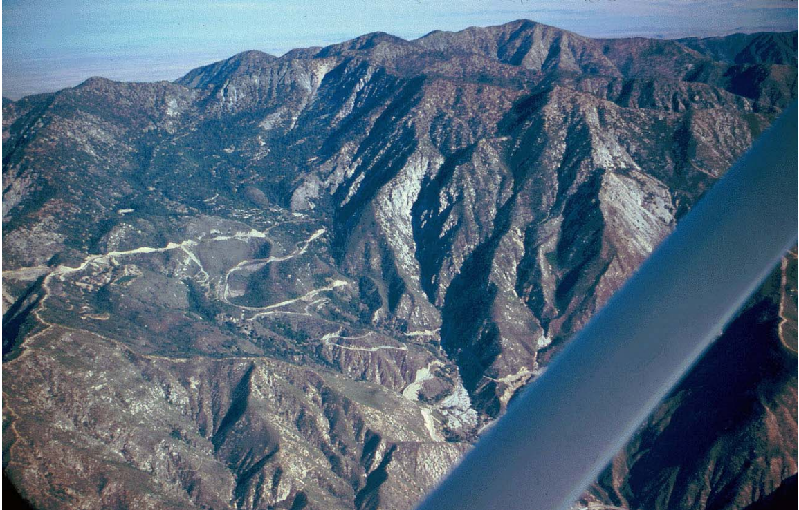
Photo 55. Crystal Lake landslide. View is to the north. Landslide fills the canyon in the left part of the photograph; switchbacks in the road are within the landslide deposit. Mount Baden Powell is the highest peak on the skyline.
