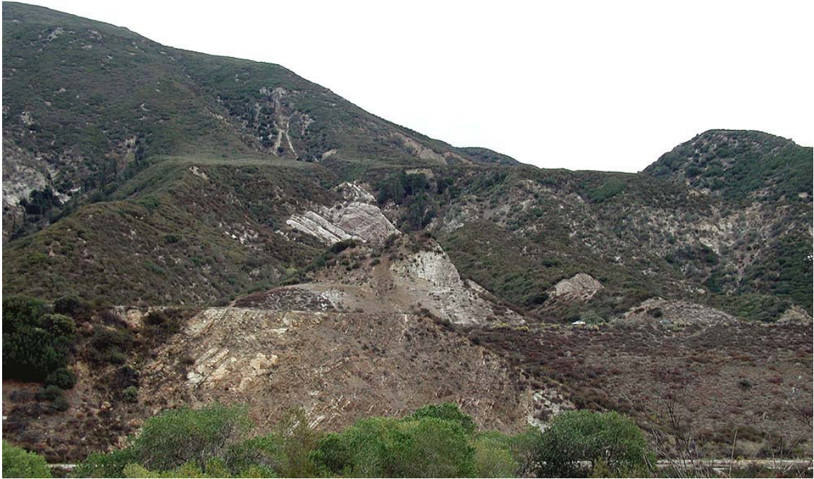
Photo 99. View looking east at Cosy Dell. North dipping Cretaceous sedimentary rocks of Cosy Dell area are exposed in road cut along old U.S. Highway 395 just beyond green trees. Top of highway cut is Interstate 15. Beyond sedimentary rocks of Cosy Dell area are south dipping thick beds of the Cajon Valley Formation (Tcv) that are overlain by old alluvial-fan deposits (Qof).
