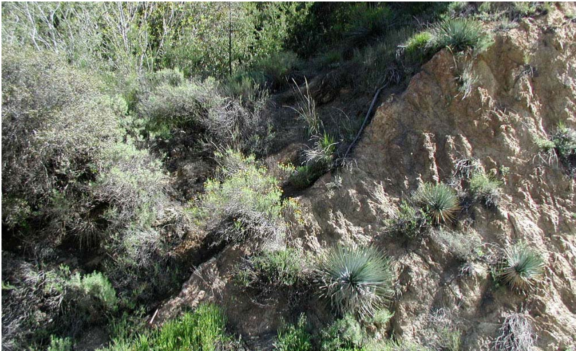
Photo 139. South Fork Lytle Creek Fault exposed along Lytle Creek Road. The pick in the lower left part of the photograph rests on the footwall of the fault. The fault zone consists of about 3 m of black gouge and finely sheared and comminuted rock (largely hidden by vegetation in this photograph).
