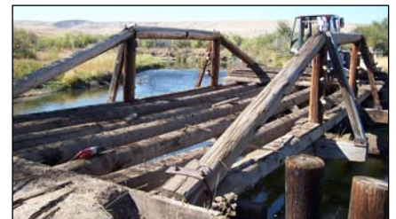
Bridge work in progress.
