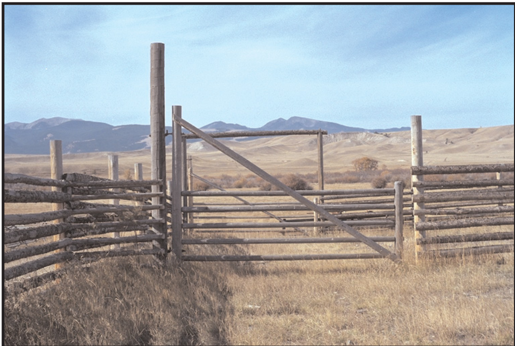
Photo 3-1-66 : (Z-12) Typical 5-Rail Braced Gate.
