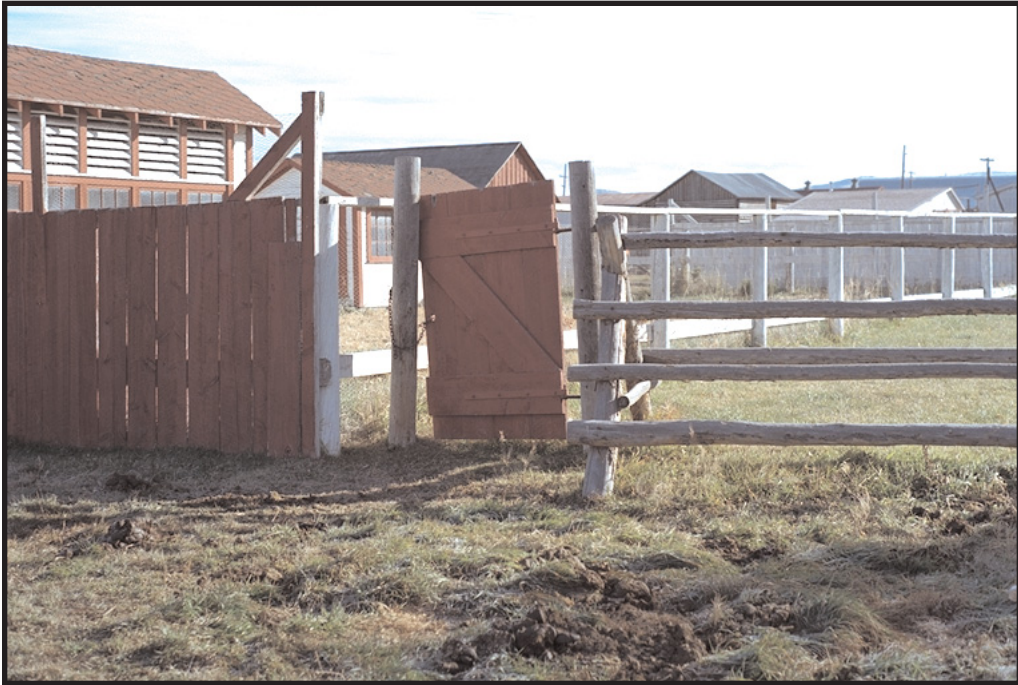
Photo 3-1-67 : (V-08) Vertical Board Gate (added by the NPS in the 1970s) with Jack-Leg Fence (right) and Vertical Board Fence (left).
