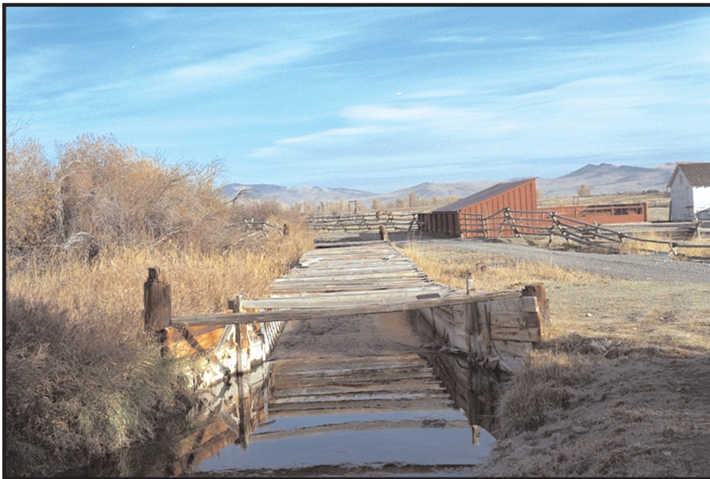
Photo 3-1-8 : (S-22) The Kohrs-Manning Ditch crosses Johnson Creek via a wooden flume (HS-50).
