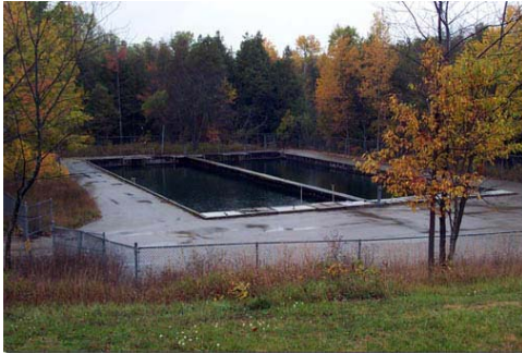
-USFWS The effluent basin at the Jordan River National Fish Hatchery settles out waste solids from fish culture operations, minimizing the impact on the Jordan River.
