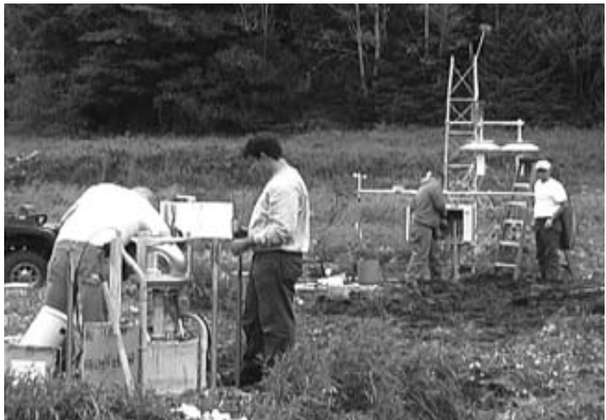
Climate tower construction
