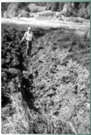
Tidal channel construction
