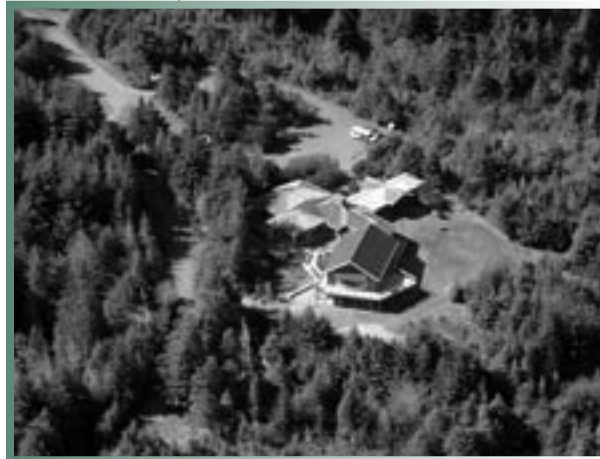
South Slough NERR Interpretive Center
