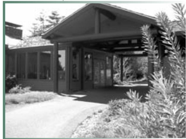
South Slough NERR Interpretive Center
