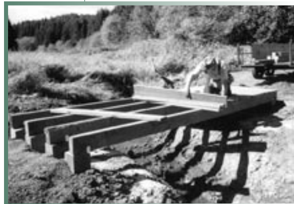
Maintenance staff constructs trail bridge
