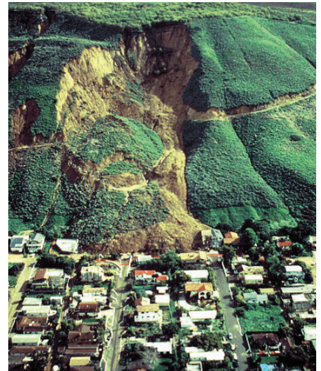
Homes lie damaged under this large earth flow in LaConchita, Calif., Saturday, March 4, 1995. On January 10, 2005, a portion of this area became a debris flow during heavy rain, destroying several homes and killing 10 people. (USGS photo/Robert L. Schuster)
