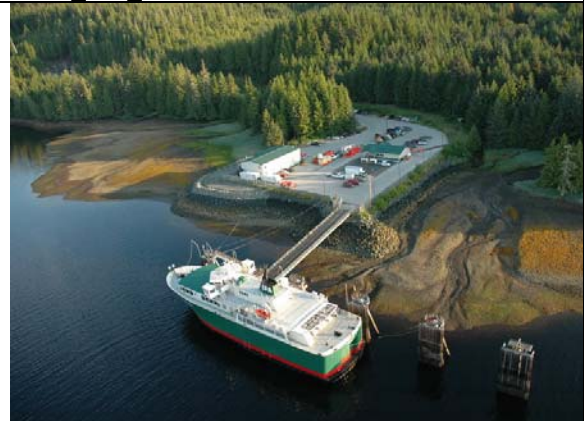
Ferry terminal near Hollis (Kasaan Bay) SE07_MM_01772
