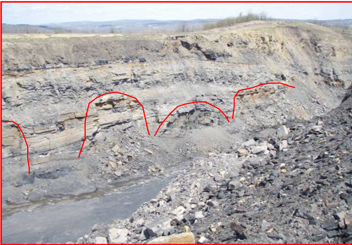
Figure 6. Concave indentations (red arcs) defined by joint-bounded blocks in sandstone overlie subsided rooms in the Pittsburgh seam. Subsidence damage extends along the highwall through the slide area.
