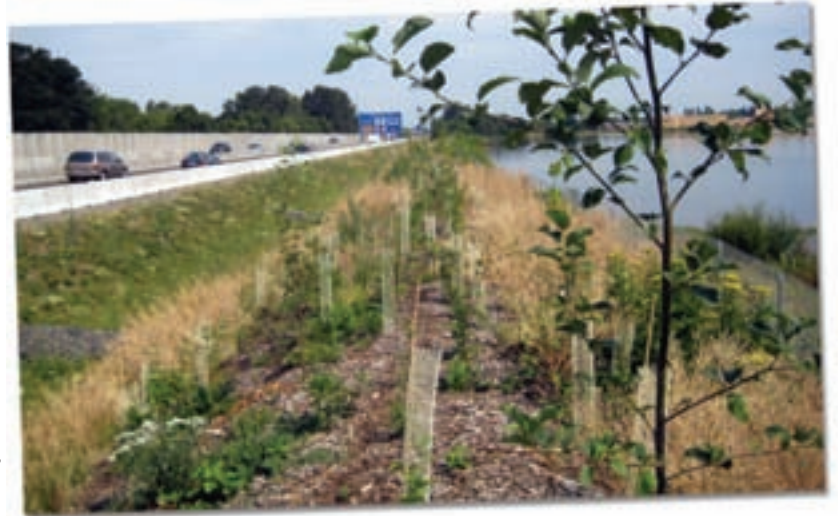
After removing trees and plants to widen seven Interstate 5 bridges in Salem, ODOT is working with Eugene-based Second Growth to plant 35,000 new trees and shrubs.
