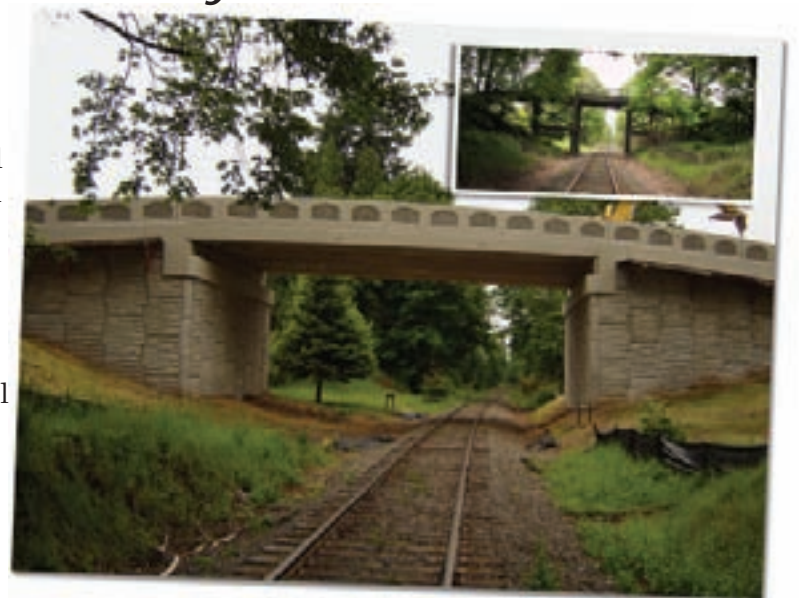
The new Portland & Western Bridge in Columbia City was noted for its design excellence. The old bridge (inset) was made of timber and in need of significant repair.
