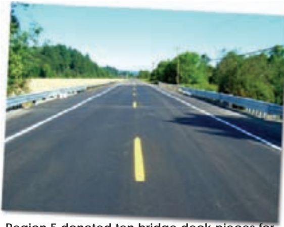
Region 5 donated ten bridge deck pieces for this completed bridge replacement project on Highway 47 in Region 1.
