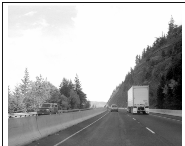
Median concrete safety barriers, like the one above, help save lives.
