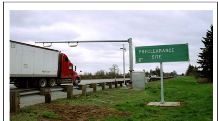
An 18-wheeler passes over weigh-in-motion scales and under transponder readers as it approaches the Woodburn port of entry on I-5.
