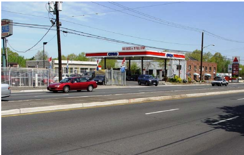
Raised curbed median near accident location.
