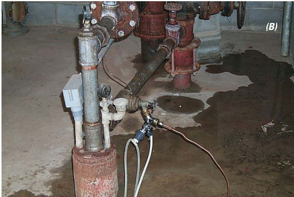
Figure 3. Connections to sample tap on discharge line (A) and at the wellhead (B).
