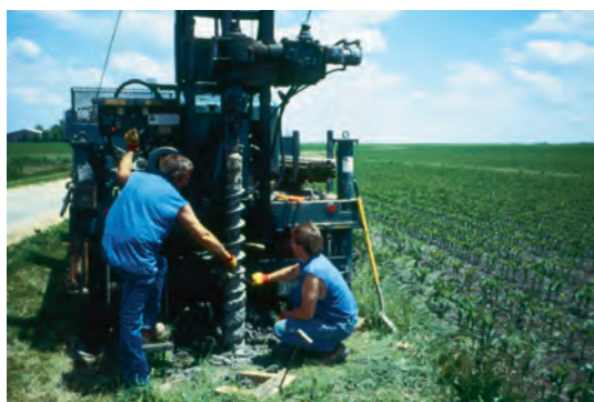
Most wells sampled for agricultural and urban land-use studies were observation wells installed by NAWQA.
