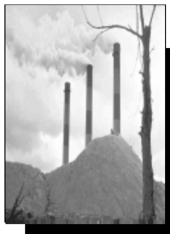
New and pending regulations will help decrease emissions from waste incinerators
