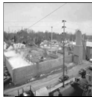
Waste Water Treatment Plants are reducing mercury discharges via voluntary pollution prevention programs
