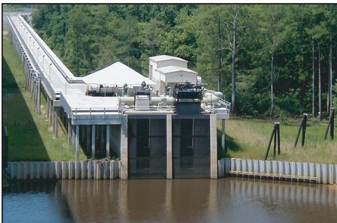
Figure 1. Ouachita River intake and pumping facility (photograph by John Czarnecki, U.S. Geological Survey).
