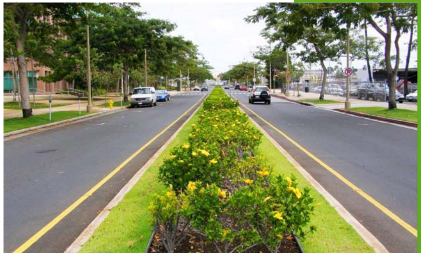
Top: Ohe Street was realigned. Below: Ilalo Street now serves as a major waterfront roadway.
