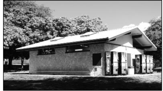
New and improved restroom facility at Diamond Head
