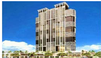
Keola La'i 63 affordable condominiums (under construction)
