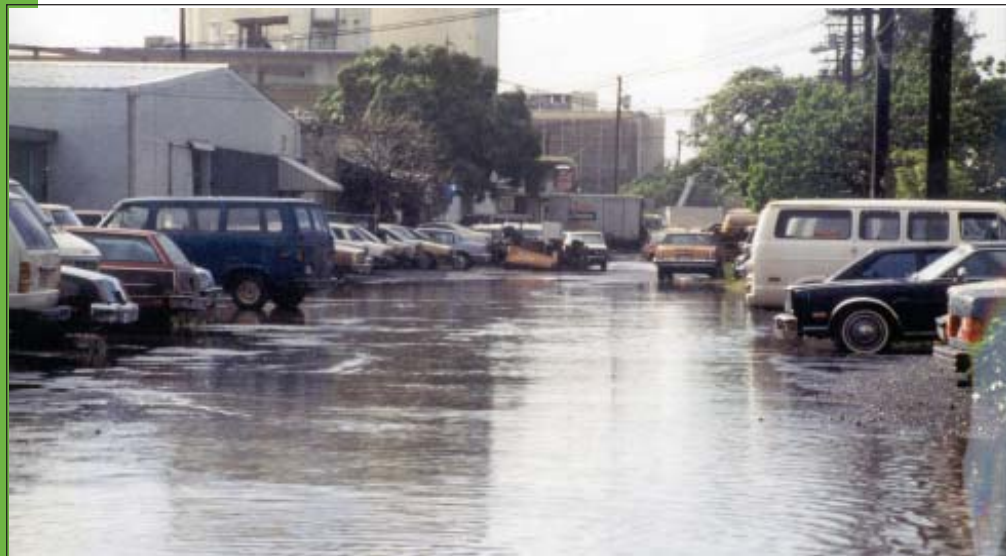
At left, current Queen Street infrastructure condition.
