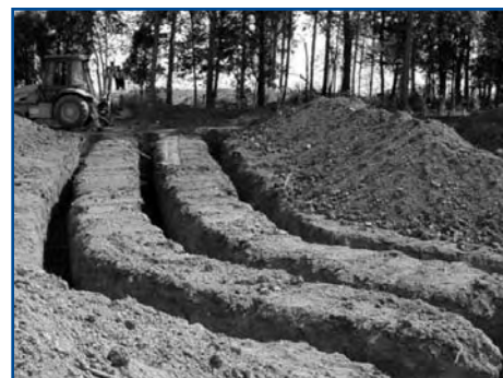
Figure 8. GHP trenches behind ZEH3.
