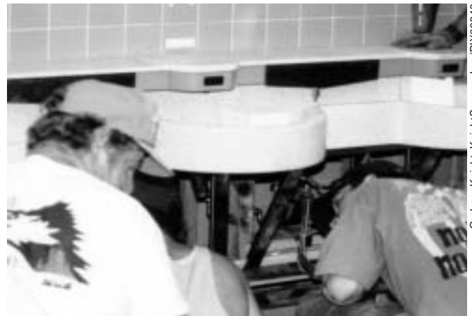
Workers make fixtures more water-efficient at the Carl Hayden Visitors Center.
