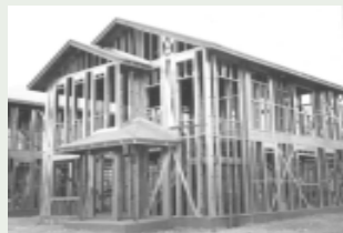
Recent steel frame project
