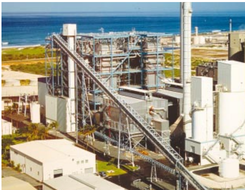
AES coal-fired power plant, Campbell Industrial Park, Oahu
