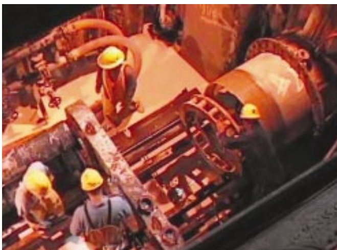
Evening work at the Nimitz Highway Microtunneling Project
