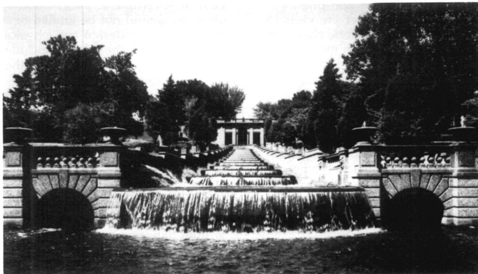
FIGURE 3 & 4: The terraced water cascade is the major design element at Meridian Hill Park in Washington, D.C., which served as a prototype for large scale and decorative usage of exposed aggregate concrete. (Photo credit: Jack E. Boucher, Historic American Building Survey [HABS])
