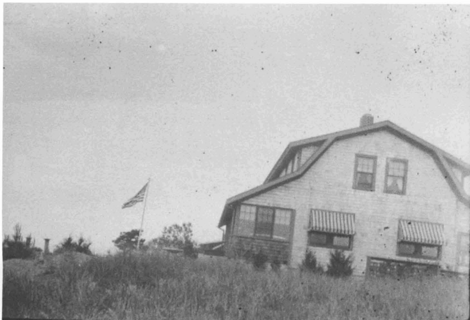
Fig. 2 Snapshot view of farmhouse from cove showing second dormer and gambrel roof, post 1931
